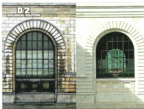
Building Façade Cleaning
